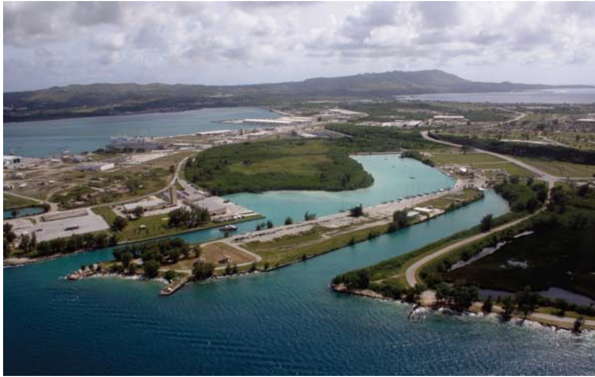
Sumay Cove Area adjacent to the Inner Apra Harbor, Guam.
