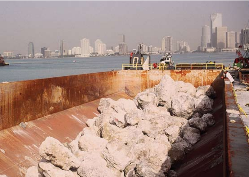
Coastal construction in Miami, FL.
