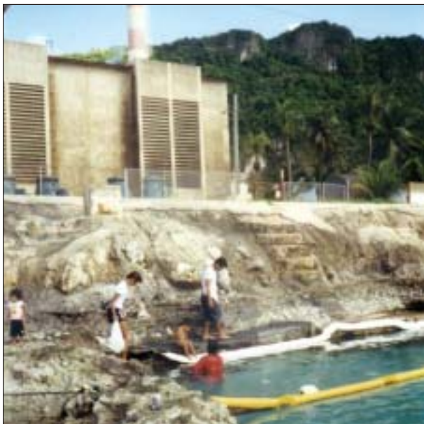
Figure 275. Guam's main power plant (Photo credit: Donna Turgeon).
